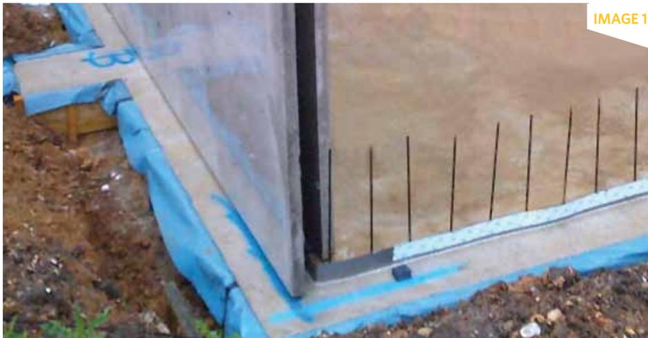
CCP designed, supplied and installed the entire basement for this contract in less than one week on site using its “double wall” precast/insitu concrete hybrid system which offers all of the advantages of precast concrete with the robustness that insitu concrete affords under the ground. As can be seen, the natural quality of finish is good enough to receive direct decoration if required. This would not be possible to achieve by any other construction method.
